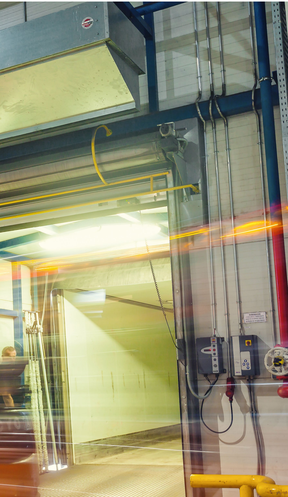
ProtecTor door air curtains effectively screen incoming cold air in the loading bay in Heineken's "Volga" subsidiary in Nizhny Novgorod in the heart of Russia.
