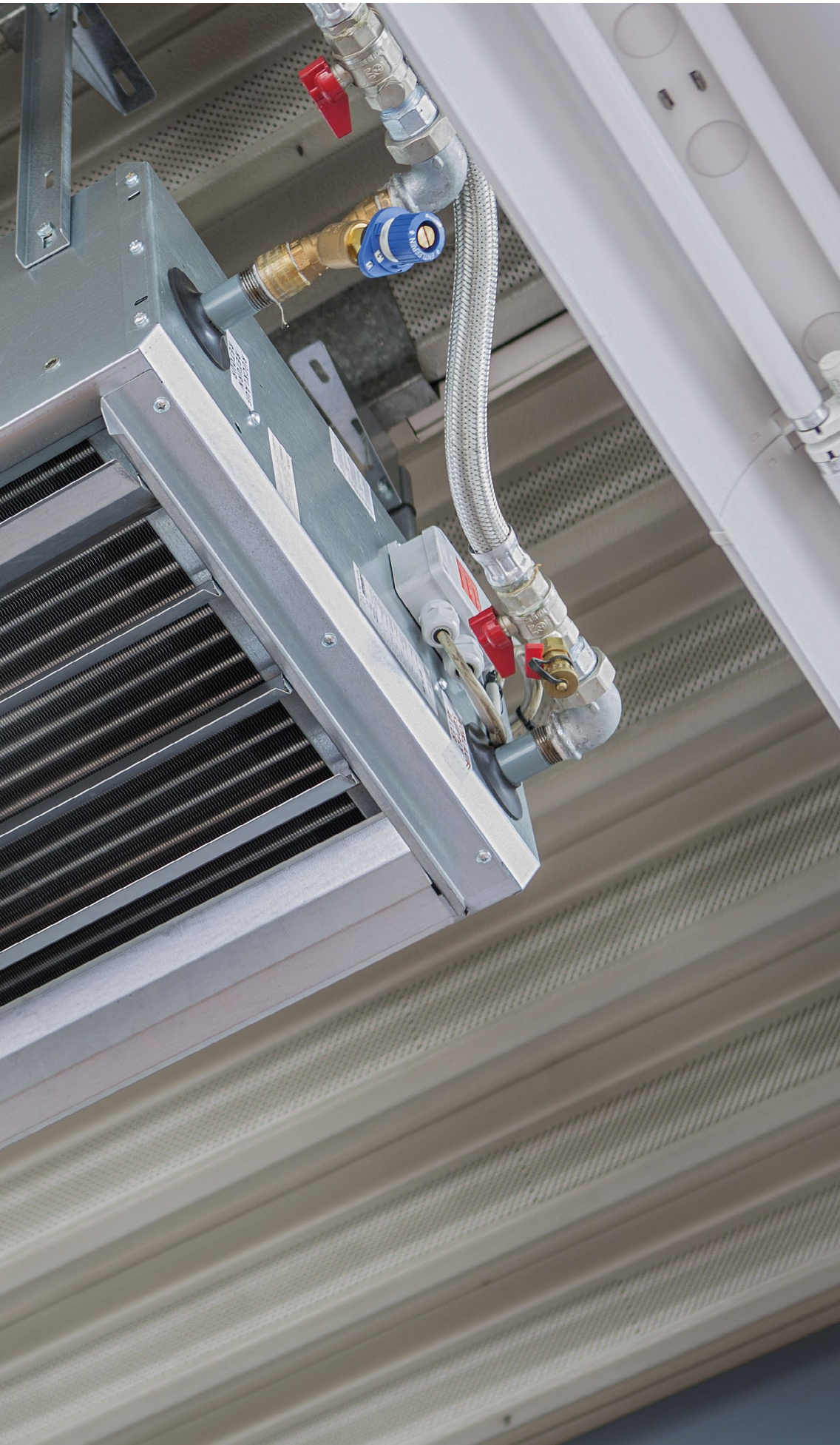
Ceiling-mounted TIP unit heaters heat the showrooms belonging to the Seyfarth car dealership in Gotha, Germany.
