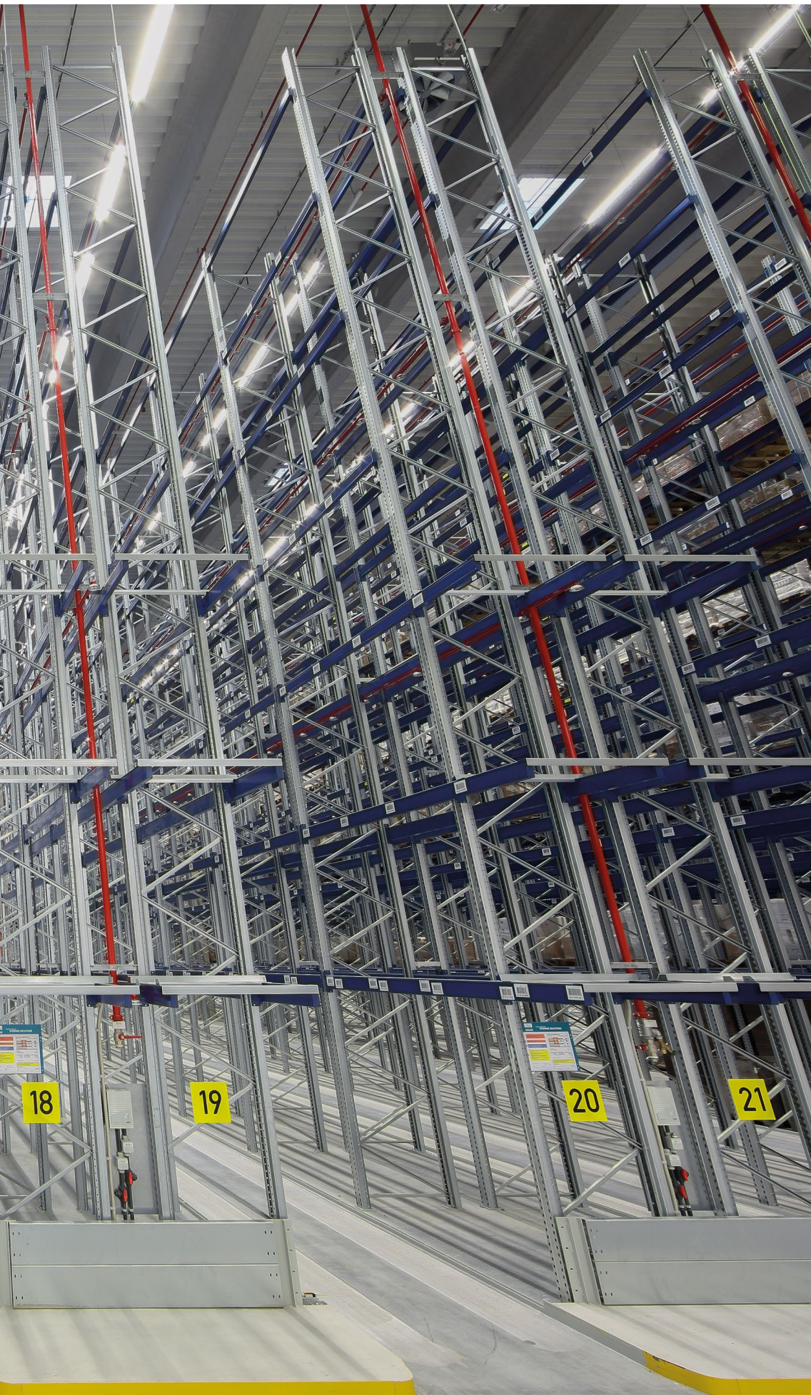
TOP unit heaters for excellent climate in the high-bay warehouse and loading area. Spedition Metzger, Neu-Kupfer, Germany
