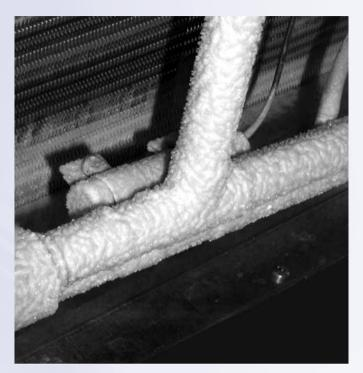
When an air-cooled heat pump is operating in heating mode, the outdoor air is relatively cool and the outdoor coil acts as an evaporator. Under certain conditions of temperature and absolute humidity, frost might form on the surface of the evaporator. This layer of frost will interfere with the operation of the heat pump by making the pump work harder and, therefore, inefficiently. The heat pump unit will "defrost" regularly when frost conditions occur.
