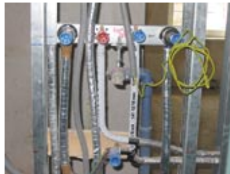
Example: Installation in partition walls in domestic areas with HERZ pipes
