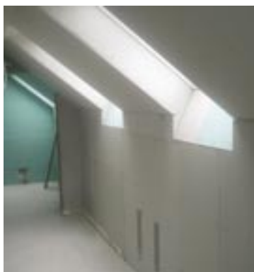
Renovation of apartments
