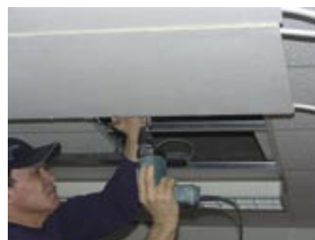
Installation of cooling ceiling
