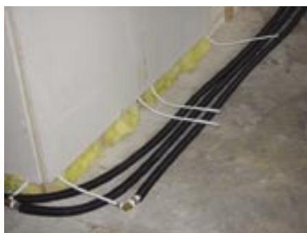
Connection of wall heating
