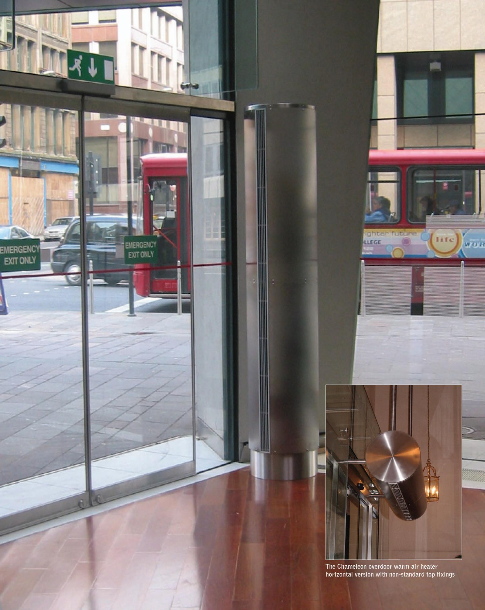
The Chameleon overdoor warm air heater horizontal version with non-standard top fixings
